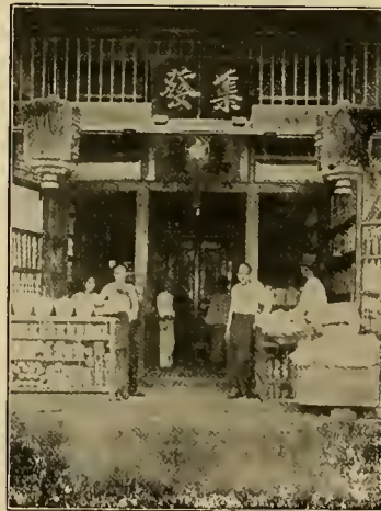
Chinese Store, lighted with a "Best" Lighting System.
